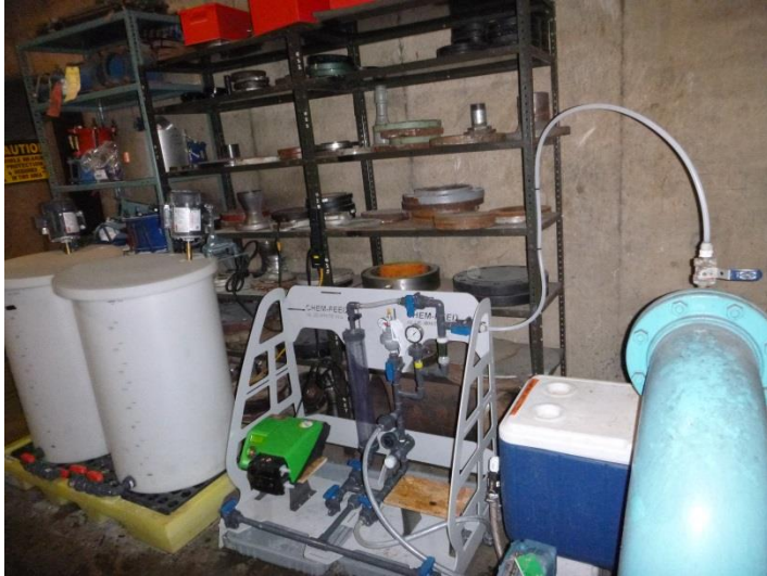
Figure 2. Zequanox Application System. Product injection occurs where flexible tube connects to port on blue pipe at center right in the photo.
