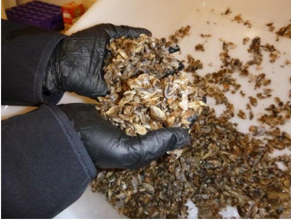
Figure 15. Mussels Removed from a Strainer Basket during Cleanout at Hoover Dam on December 5, 2013.
