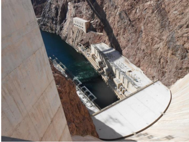
Figure 13. Post Treatment Picture of Tailrace Taken from the Top of Hoover Dam. Bubbles are visible adjacent to motoring units (untreated) at center of picture. No foam residue visible from the recently completed Zequanox treatment.
