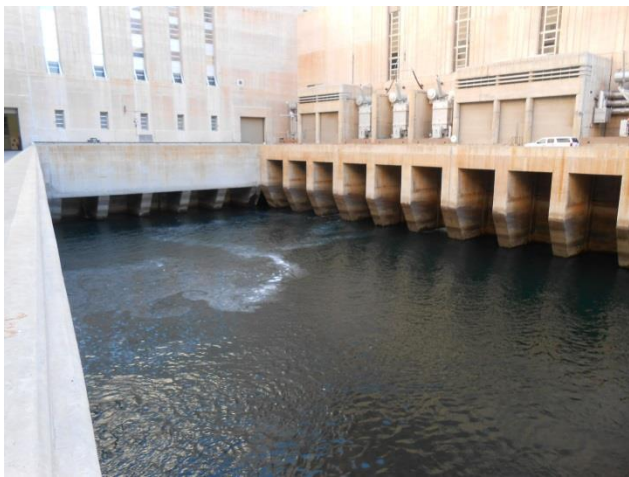
Figure 11. Discharge Water Exiting Hoover Dam during a Zequanox Treatment. Foam visible at center of image is adjacent to discharge of cooling water system treated with Zequanox.
