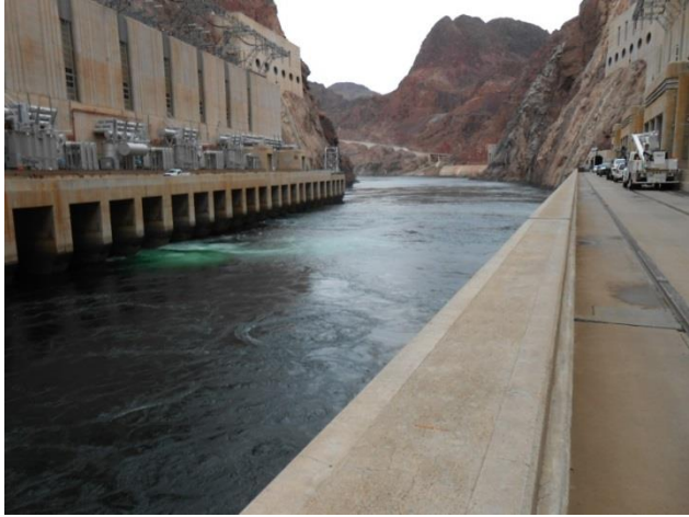
Figure 10. Discharge Water Exiting Hoover Dam from a Unit Not Treated with Zequanox. Visible bubbles from an untreated unit visible as white area in the water just left of center in the photo.
